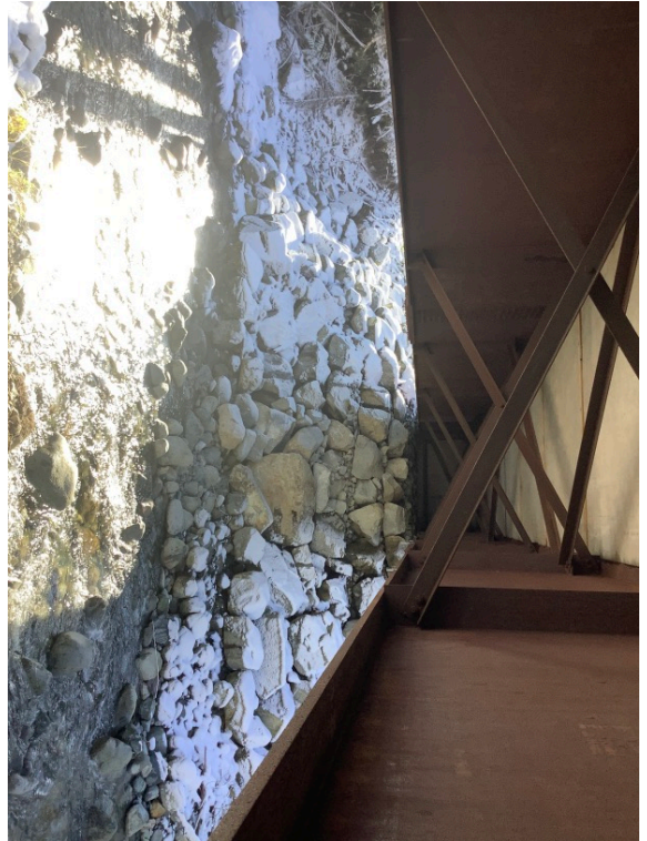
Right Bank Abutment when facing downstream
