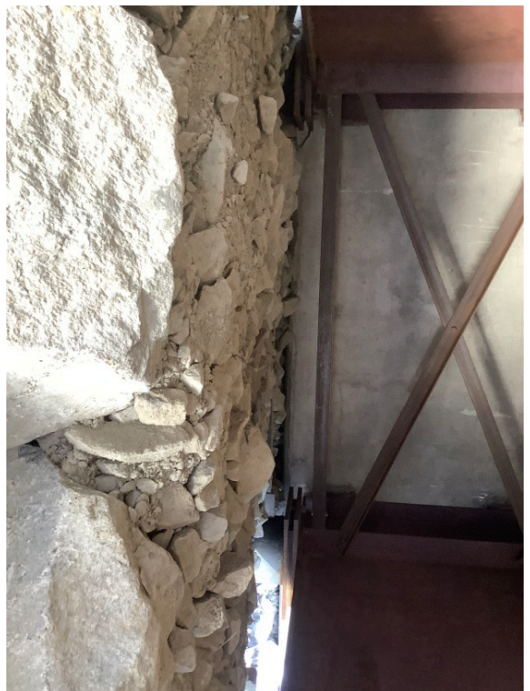
Right Bank Abutment when facing downstream
